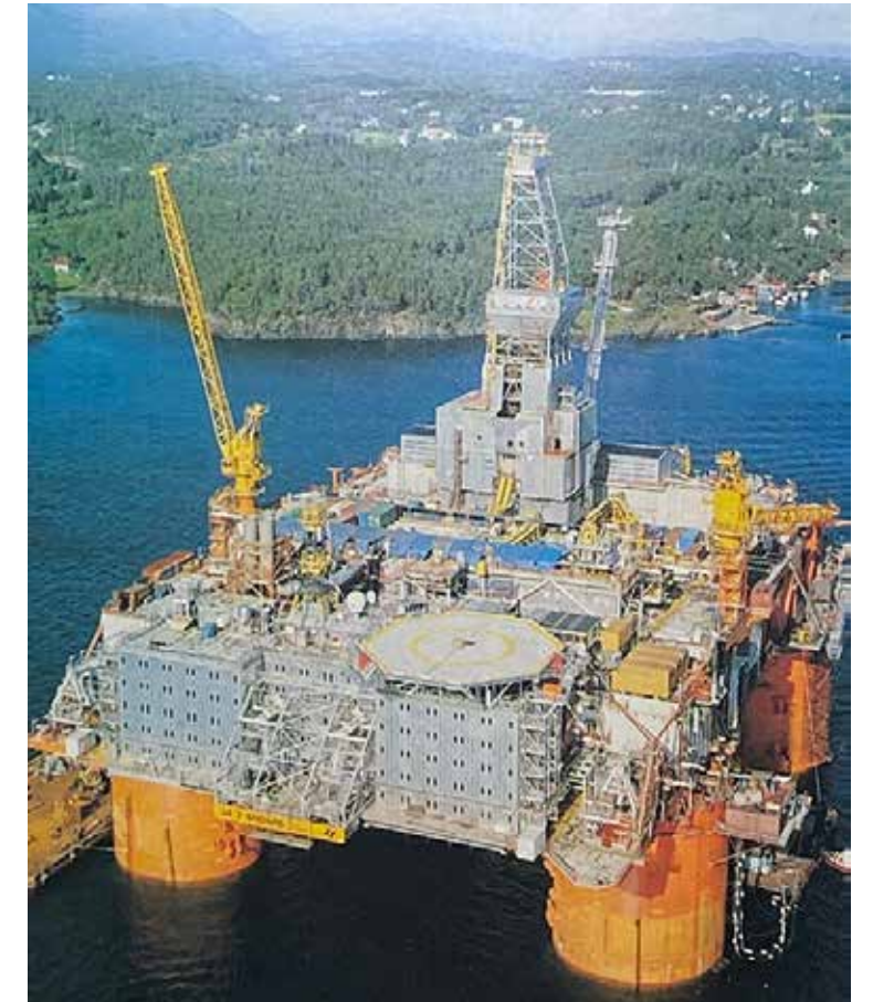
Snorre 1992 The Snorre TLP near Stavanger ready to be towed onsite.
