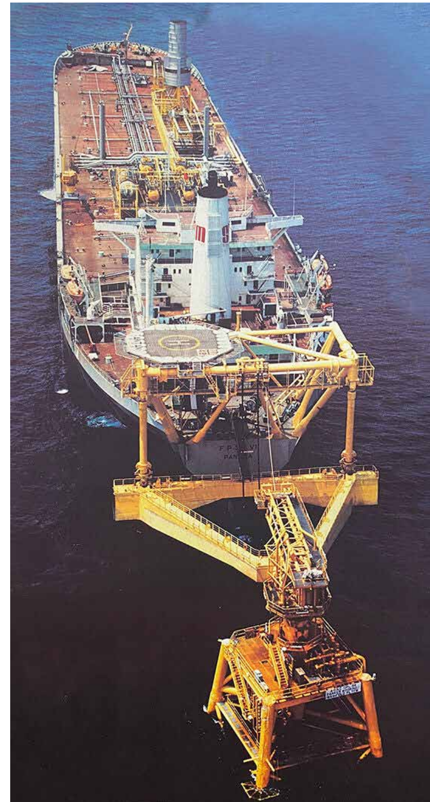
Installed in 1985, this jacket/soft yoke combination was build by SBM for Ashland Oil and Gas in 135ft of Nigerian waters. It could store 1.75 million barrels of processed oil.
